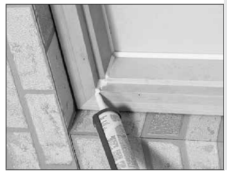
FIGURES 26 and 27: Caulk the jamb and the exterior trim.
