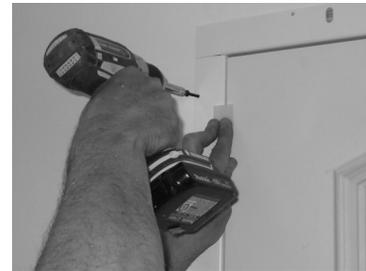
**5.** Close door and secure strike jamb using a 1/8" spacer to obtain a consistent gap as you work toward the bottom. Install remaining screws in header.
