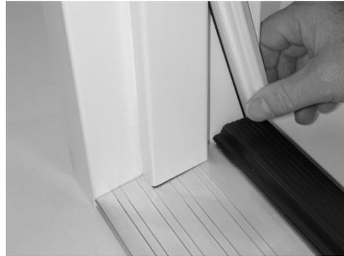
12. If K2A, Pull weather-strip out of the kerf near sill to allow room for caulking. Install sill extender if required.
