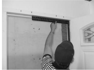
**4.** Remove pre-hang clip and open door. Use a carpenter's square to square header to hinge jamb. Install one drywall screw in center of header.
