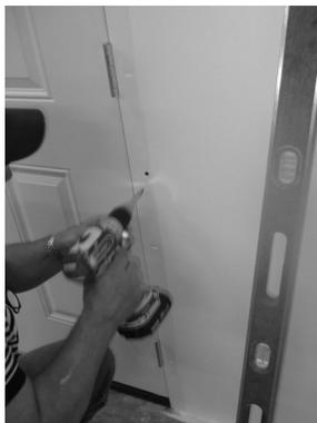
**3.** Install the remaining screws in the hinge jamb starting at top, checking for plumb as you work toward the bottom.
