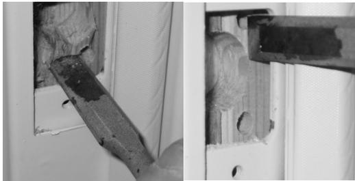
10. Clear out the remaining wood with a wood chisel.
