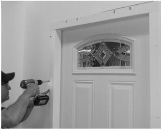
8. Secure the header closure trim and jamb closure trim near the top corners first to maintain a tight square fit in the corners. Properly installed closure trim does not narrow into the opening or spread apart allowing for unsquared condition to the wall. Insert the remaining screws. 6 screws per each vertical closure trim and 3 per header closure trim.
