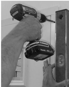
**2.** Use a level to plumb hinge jamb. Secure near top corner with a drywall screw.
