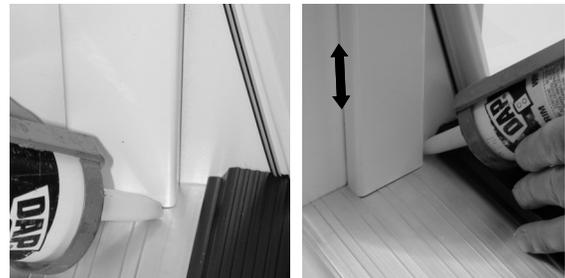
13. Use a high quality latex caulk to seal all gaps between jambs and sill. Allow caulk to set before reinserting weather-strip. Also caulk the outside of sill and closure trim to floor. For exterior applications caulk frame to closure trim at both jambs and header, as indicated by arrow above.
