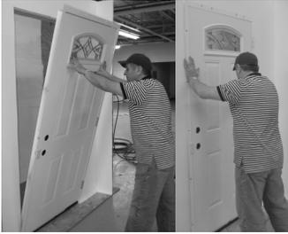
**1.** Place bottom of door assembly in bottom of opening. Lean top of door away from wall. Have a helper caulk bottom of sill. Stand door upright, centered in opening and against wall.
