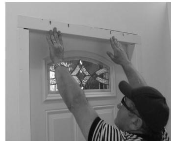
**7.** Slide header closure trim into header. Adjust vertical and header closure trims to obtain a good fit in the top corners.
