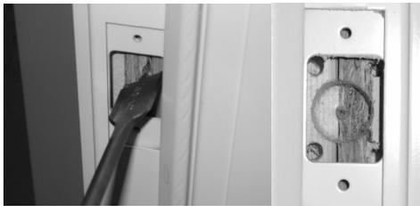
9. Prepare stud for deadbolt clearance. Bore a 7/8"-1" hole to a depth of 1" from rabbet of frame. Drill a 3/8" dia. hole at each corner to a depth of 1" from rabbet of frame.
